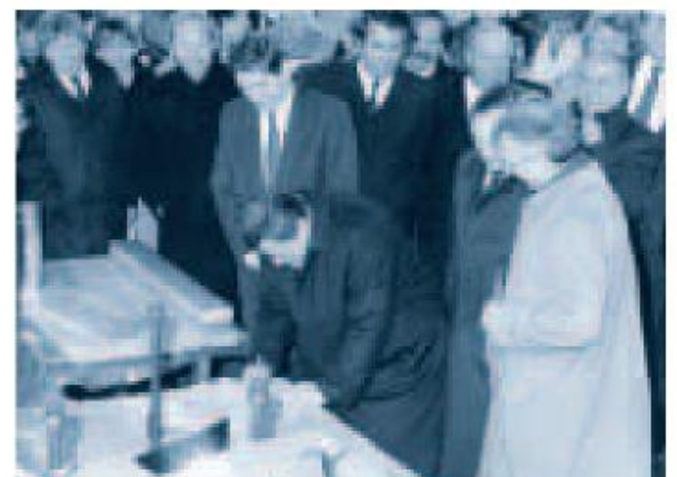
Franz-Josef Strauß laying the foundation stone.
