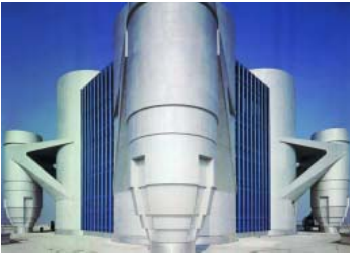
The sturdy retaining structure has the cylinders firmly in its grip.
